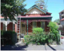
carlton north park street carlton north park street 456
