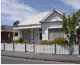
richmond miller street richmond miller street 3
