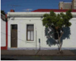
collingwood palmer street collingwood palmer street 54
