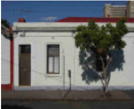
collingwood palmer street collingwood palmer street 54
