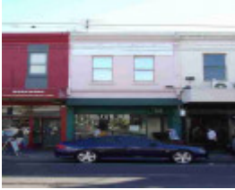
cremorne church street cremorne church street 462
