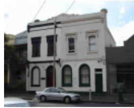
Collingwood Johnston Street 100-102.JPG
