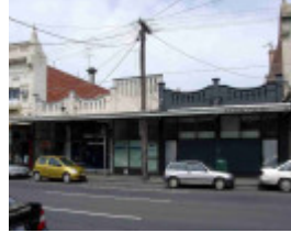
Collingwood Johnston Street 105-113.JPG
