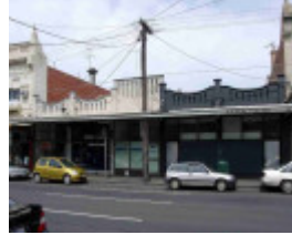
Collingwood Johnston Street 105-113.JPG
