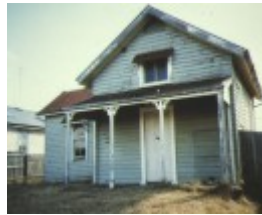
1 balmoral court house glendining road balmoral entrance feb1986
