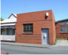
collingwood campbell street collingwood campbell street 5-11
