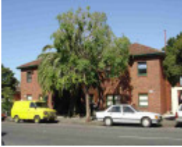
richmond lennox street richmond lennox street 180 unit 1-12
