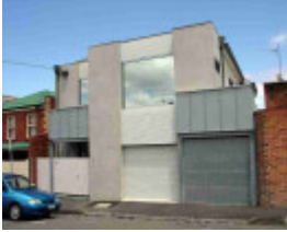
richmond dando street richmond dando street 4
