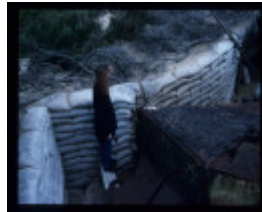
FORT NEPEAN GUN EMPLACEMENT EXCAVATION
