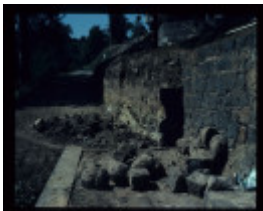
FORT NEPEAN GUN EMPLACEMENT EXCAVATION
