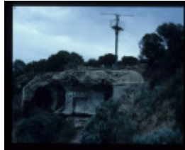
FORT NEPEAN GUN EMPLACEMENT EXCAVATION
