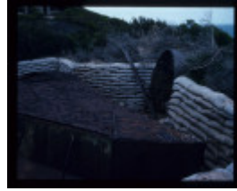
FORT NEPEAN GUN EMPLACEMENT EXCAVATION
