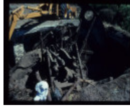
FORT NEPEAN GUN EMPLACEMENT EXCAVATION
