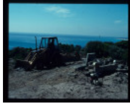
FORT NEPEAN GUN EMPLACEMENT EXCAVATION
