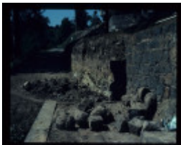
FORT NEPEAN GUN EMPLACEMENT EXCAVATION
