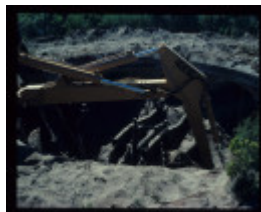
FORT NEPEAN GUN EMPLACEMENT EXCAVATION
