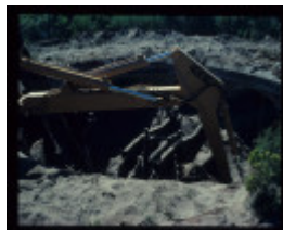
FORT NEPEAN GUN EMPLACEMENT EXCAVATION
