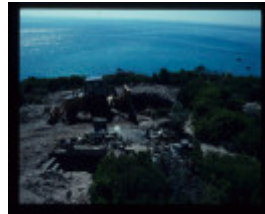
FORT NEPEAN GUN EMPLACEMENT EXCAVATION
