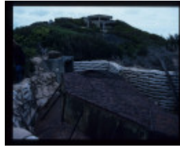
FORT NEPEAN GUN EMPLACEMENT EXCAVATION
