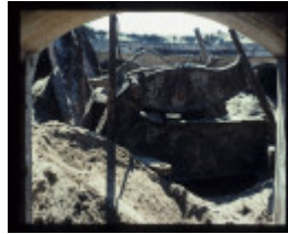
FORT NEPEAN GUN EMPLACEMENT EXCAVATION
