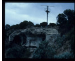
FORT NEPEAN GUN EMPLACEMENT EXCAVATION
