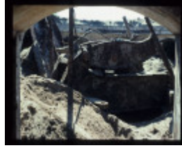
FORT NEPEAN GUN EMPLACEMENT EXCAVATION
