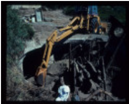
FORT NEPEAN GUN EMPLACEMENT EXCAVATION
