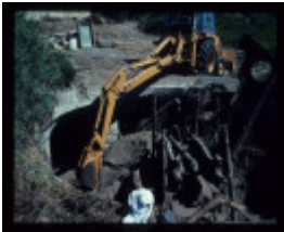
FORT NEPEAN GUN EMPLACEMENT EXCAVATION
