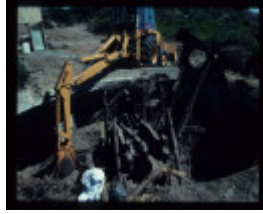
FORT NEPEAN GUN EMPLACEMENT EXCAVATION
