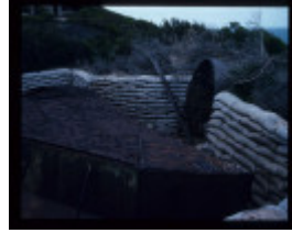
FORT NEPEAN GUN EMPLACEMENT EXCAVATION
