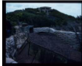
FORT NEPEAN GUN EMPLACEMENT EXCAVATION
