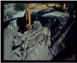
FORT NEPEAN GUN EMPLACEMENT EXCAVATION
