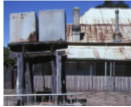
day's flour mill complex murchison corrugated iron building
