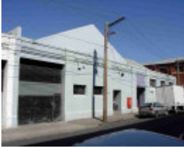
collingwood down street collingwood down street 2-4
