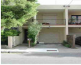
richmond egan street richmond egan street 38 unit 1
