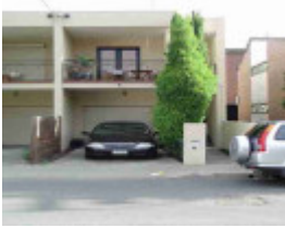
richmond egan street richmond egan street 38 unit 2
