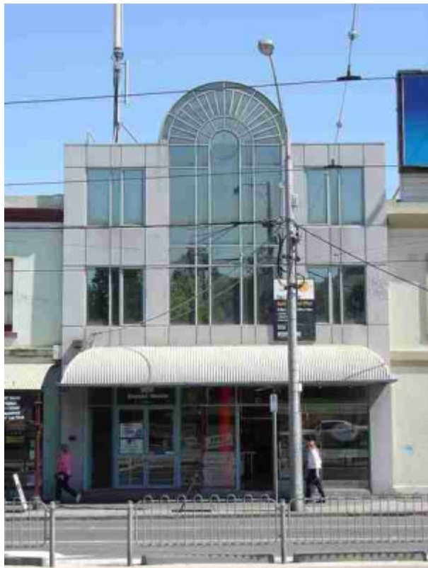
richmond bridge road richmond bridge road 2-4 unit 1-10
