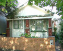
burnley bendigo street burnley bendigo street 65
