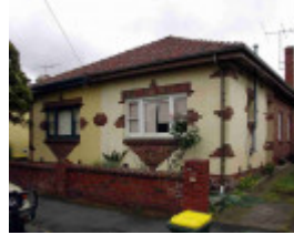
Richmond Charlotte Street 13-15.JPG
