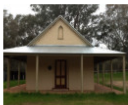
After Photograph - Reference F3875 2016
