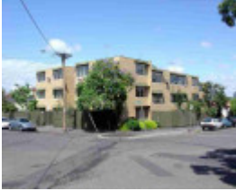
richmond docker street richmond docker street 2-6 unit 1
