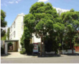
richmond docker street richmond docker street 7
