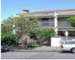
richmond docker street richmond docker street 18
