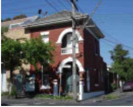
richmond lennox street richmond lennox street 227
