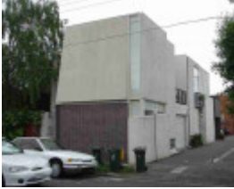
richmond brighton street richmond brighton street 146
