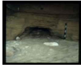
QUARANTINE STATION LIME KILN 1
