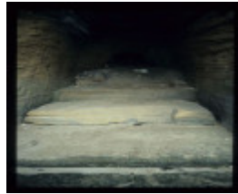
QUARANTINE STATION LIME KILN 1
