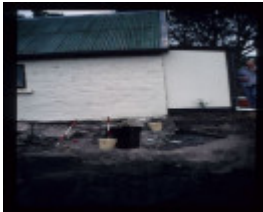
LIMESTONE COTTAGE EXCAVATION
