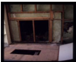
LIMESTONE COTTAGE FEATURE
