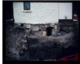
LIMESTONE COTTAGE EXCAVATION
