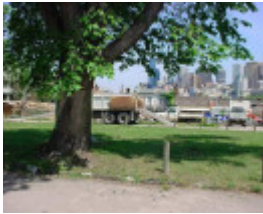
h02009 js demolition 10 nov 2003
