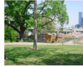
h02009 js 10 nov 2003 southern elm during demolition
