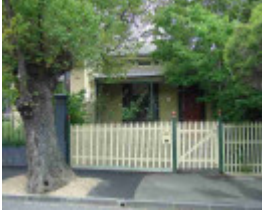
richmond clifton street richmond clifton street 17-17a
