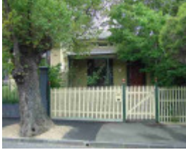
richmond clifton street richmond clifton street 17-17a
