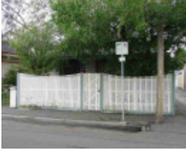
richmond cotter street richmond cotter street 22
