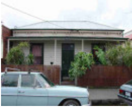
richmond cotter street richmond cotter street 25
