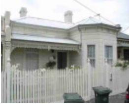
richmond cotter street richmond cotter street 28
