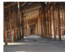
Murtoa Grain Store interior Nov 08 01
