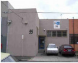
collingwood down street collingwood down street 55
