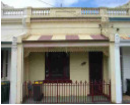
carlton north drummond street carlton north drummond street 558
