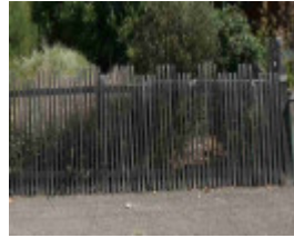
Fence - 123-125 Arnold Street
