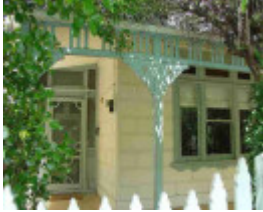
richmond alfred street richmond alfred street 13
