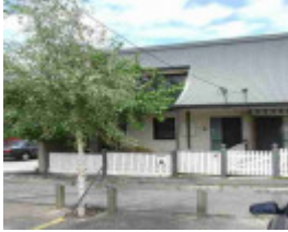
richmond allowah terrace richmond allowah terrace 10b
