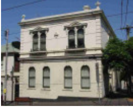
richmond church street richmond church street 384
