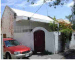
richmond loughnan street richmond loughnan street 4
