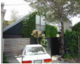
richmond loughnan street richmond loughnan street 5
