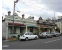
Richmond Brighton Street 122-130.JPG
