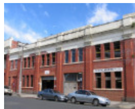
Rear of 7 Stanley Street
