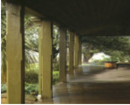
1 elderslie barringo new gisborne view of verandah
