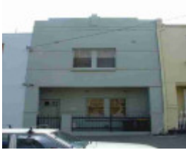
carlton north drummond street carlton north drummond street 695
