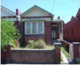
carlton north amess street carlton north amess street 161
