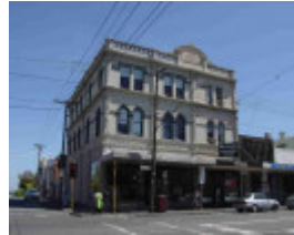
Richmond Bridge Road 130- 132A.JPG
