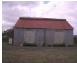
new gisborne railway station complex station road goods shed apr1995
