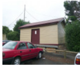
NEW GISBORNE RAILWAY STATION COMPLEX SOHE 2008
