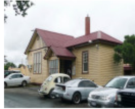
NEW GISBORNE RAILWAY STATION COMPLEX SOHE 2008
