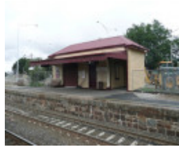
NEW GISBORNE RAILWAY STATION COMPLEX SOHE 2008
