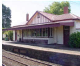
Gisborne Station Building
