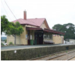
NEW GISBORNE RAILWAY STATION COMPLEX SOHE 2008
