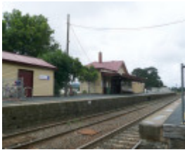
NEW GISBORNE RAILWAY STATION COMPLEX SOHE 2008
