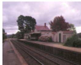
new gisborne railway station complex station road trackside view apr1995
