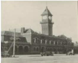
Richmond Town Hall (on Bridge Road) before major renovations. Published in City of Richmond, Report of the Council 1924-25.
