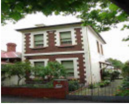
richmond elm grove richmond elm grove 12
